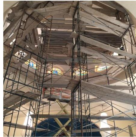
We are in the midst of nearing completion of the dome work. It is in the paint stage at this time, and anticipate completion by the end of next week, with scaffolding still onsite. The sealing of the brick is complete. The outside restoration of the wood doors is still in progress. The work that will commence after the completion of the dome is; the painting of the ceiling, complete cleaning of the church, installation of the new carpeting, and the re-installing the pews.
